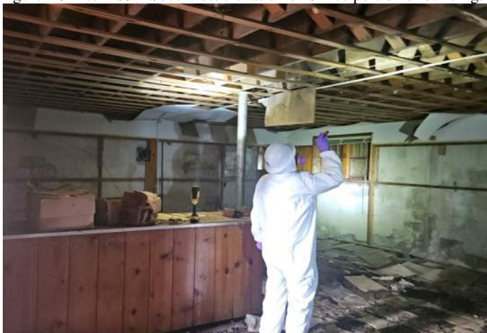
Figure A5 - Item S1, S2 – Floor Framing and Foundation Walls of Office Wing.
