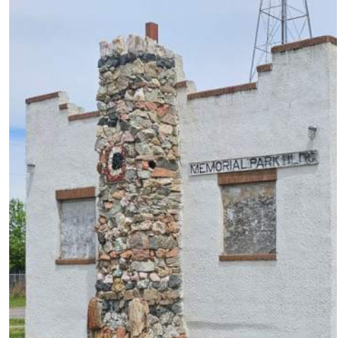
Figure 8: View of the west wall of the Office portion of the building showing the existing stone chimney wall, the stones of which are recommended to be salvaged for future building reconstruction.
