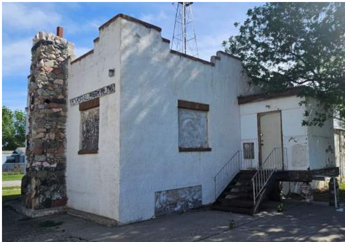
Figure A3 - Item S3 – Southwest elevation of Office portion of building.
