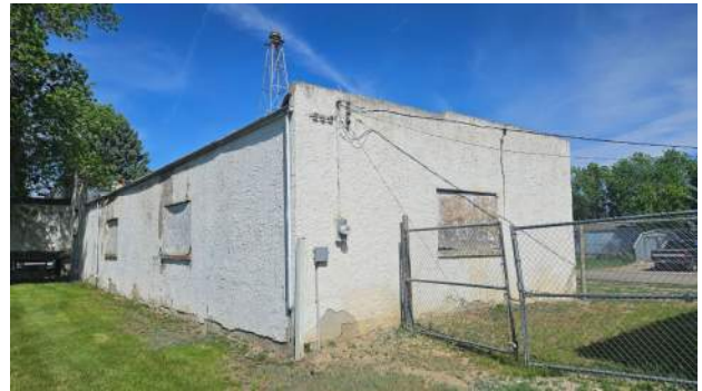
Figure B2 - Item S3 – Southeast elevation of Shop portion of building.
