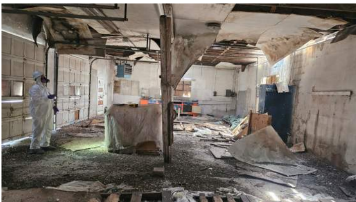
Figure B5 - Item S4 – Typical roof framing at Shop portion of building.
