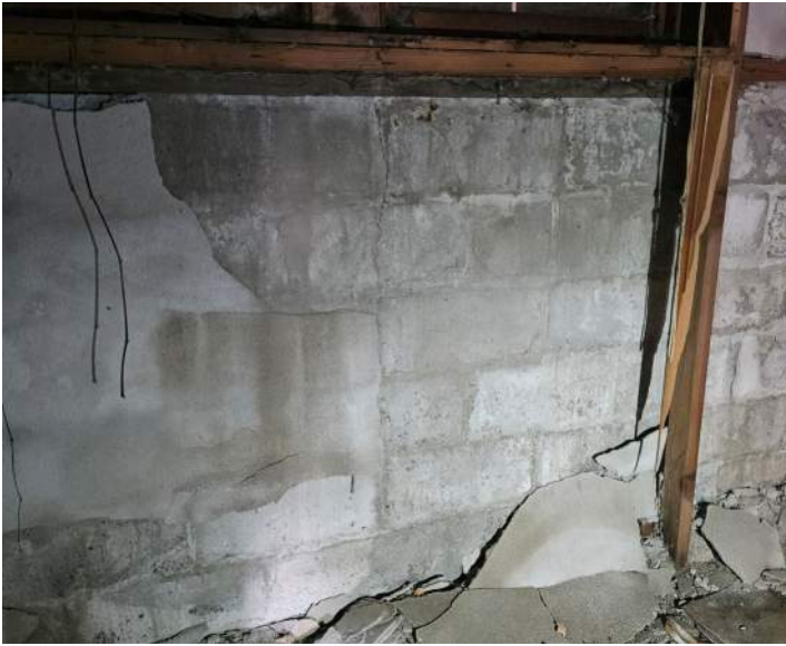
Figure A7 - Item S1 – Hollow, unreinforced Foundation Walls of Office Wing.
