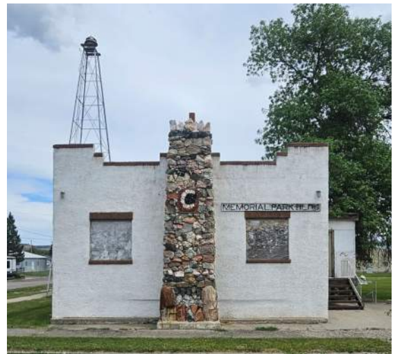
Figure A4 - Item S3 – West elevation of Office portion of building.
