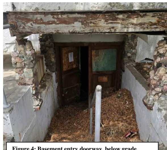
Figure 4: Basement entry doorway, below grade. Concrete stairs protected by concrete earth retaining walls serve as the access for this doorway.
