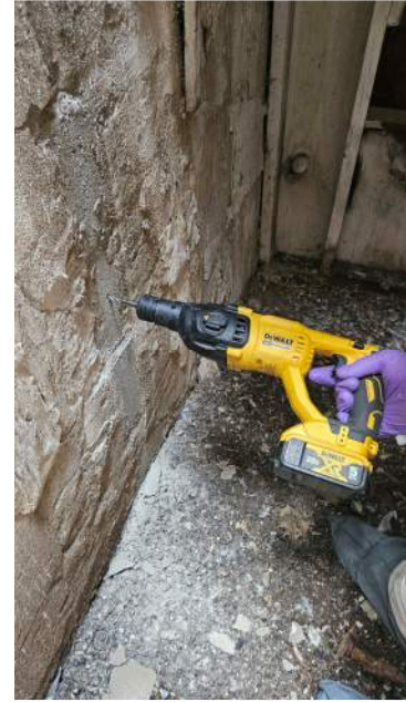
Figure A8 - Item S1 – Drilling the hollow CMU Foundation Walls of Office Wing.
