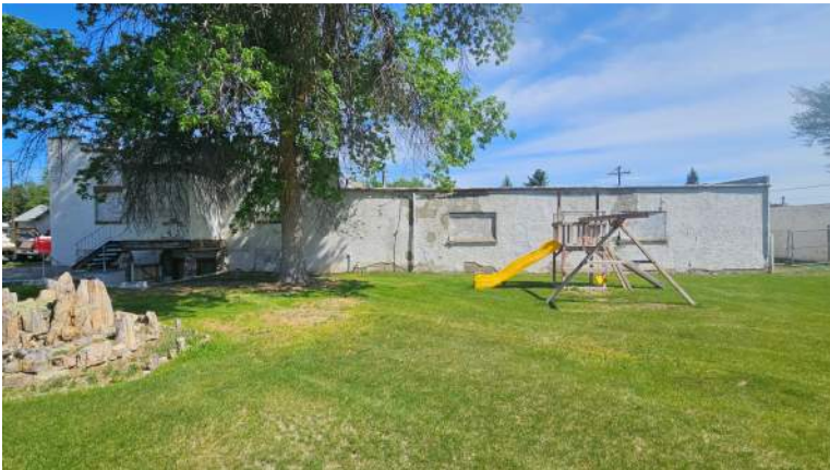
Figure B3 - Item S3 – South elevation of Office and Shop portion of building.
