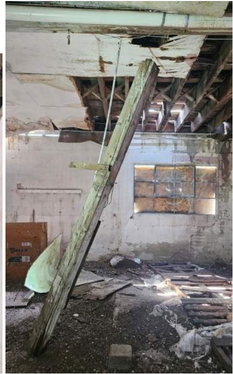
Figure 11a: (Left) View of charred Shop rafters at the northeast corner of the building; 11b (Right) View of failed roof beam support post of the Shop Wing, looking south; partial roof decking collapse/failure throughout.
