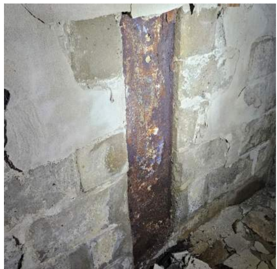
Figure 6b: Office floor steel beam support column within exterior CMU wall - Note significant steel corrosion.
