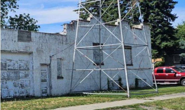
Figure A1 - Item S3 – North elevation of Office portion of building.
