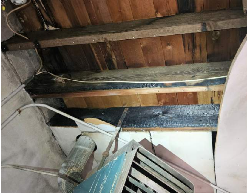
Figure 11a: (Left) View of charred Shop rafters at the northeast corner of the building; 11b (Right) View of failed roof beam support post of the Shop Wing, looking south; partial roof decking collapse/failure throughout.
