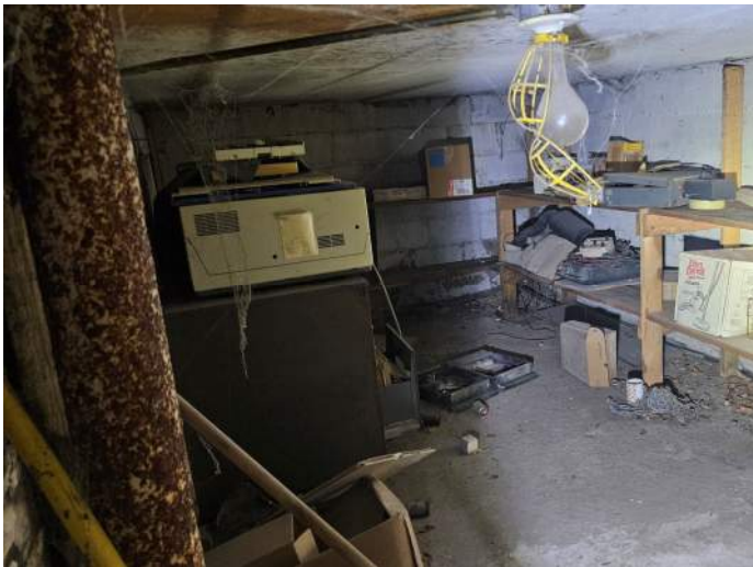
Figure A13 -Item S1, S2 – Low-headroom storage space at east side of Office wing, beneath west portion of Shop Floor.
