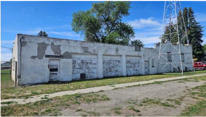
Figure B1 - Item S3 – North elevation of Shop and Office portion of building
