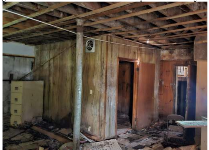
Figure A6 - Item S1, S2 – Floor Framing and Foundation Walls of Office Wing.
