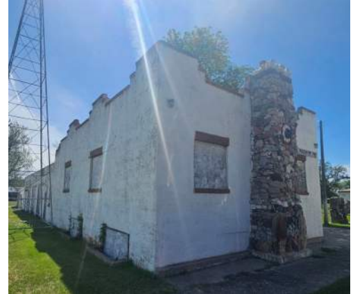
Figure A2 -Item S3 – Northwest elevation of Office portion of building.
